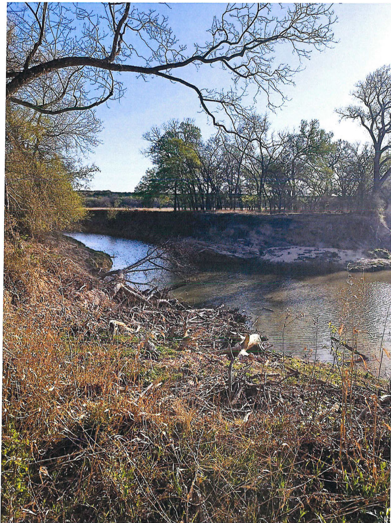
Photo 3: (Reach B-B') Downstream Limit B' Looking Upstream
