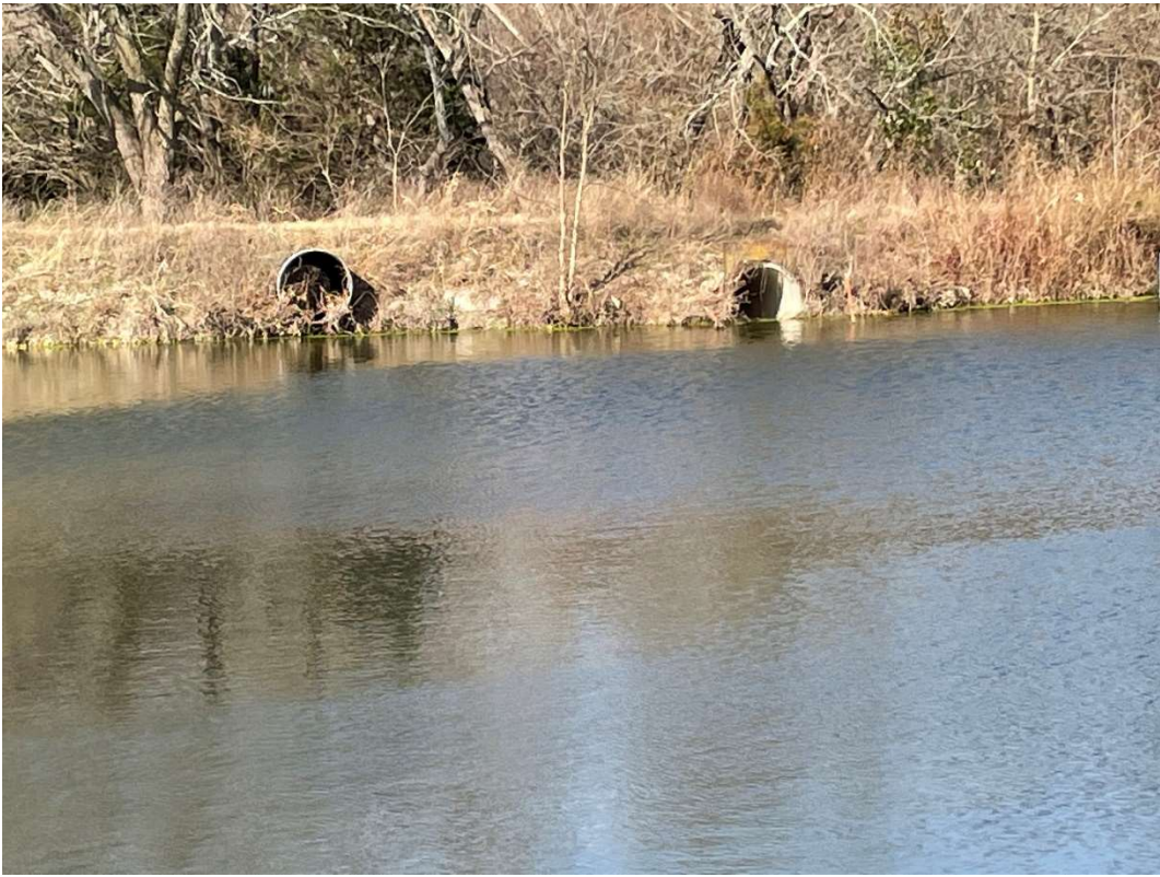
11-DAM WITH 2-18" SPILLWAY PIPES
