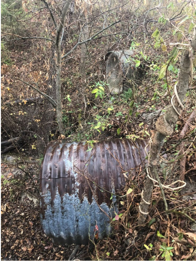
12-DOWNSTREAM END OF SPILLWAY PIPES
