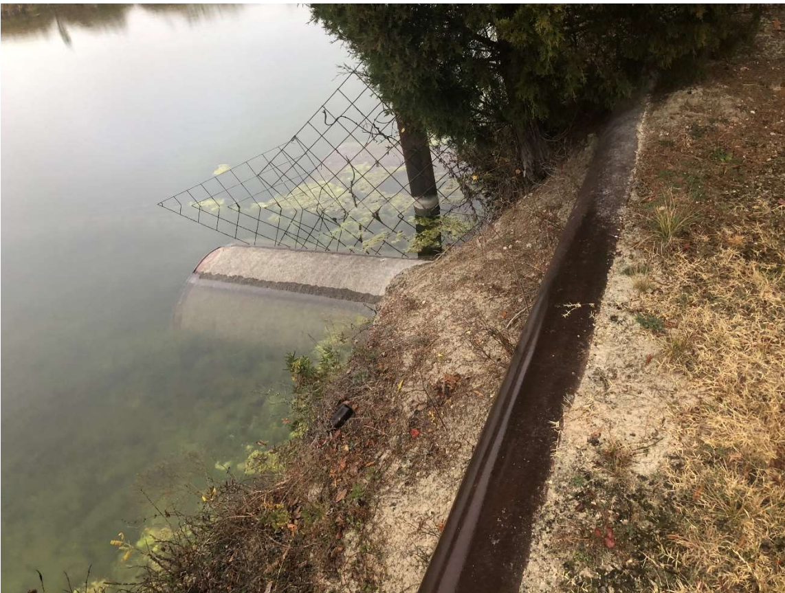
8- RCP DOWNSTREAM OF ROAD BETWEEN PONDS
