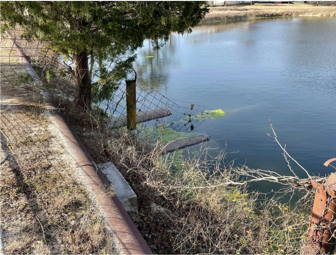
7-DOUBLE 48 INCH RCP BETWEEN TWO PONDS
