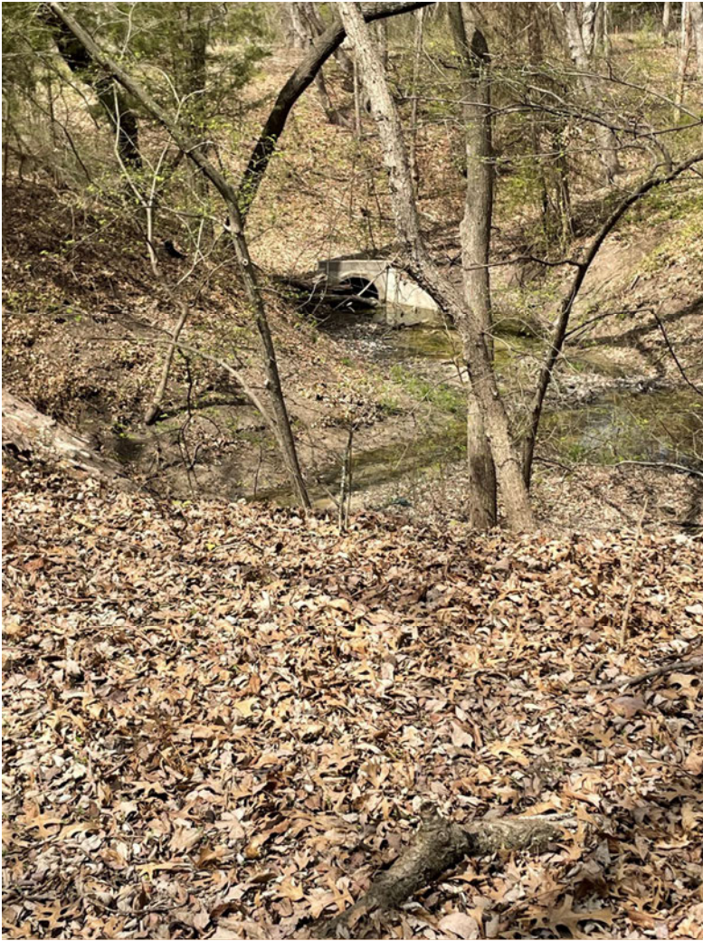
15-NEAR W PROP LINE, UPSTREAM END OF CULVERT
