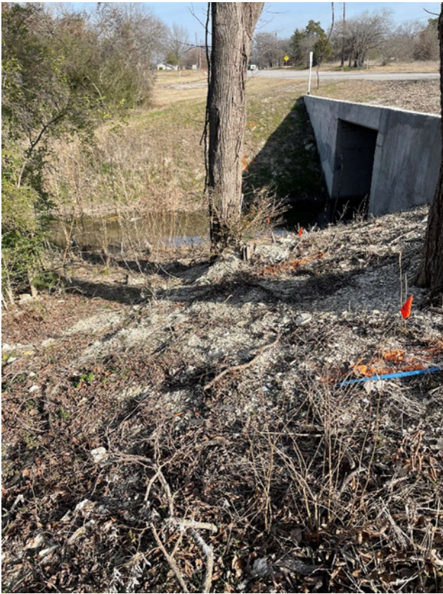
1-CULVERT ON WEST/DOWNSTREAM SIDE OF S POWELL
