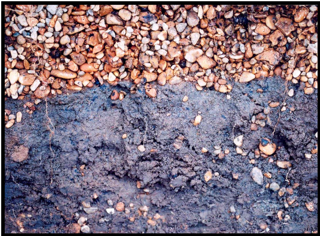
Figure 2.23 Closer View of Biological Growth at Bottom of Trench 9
