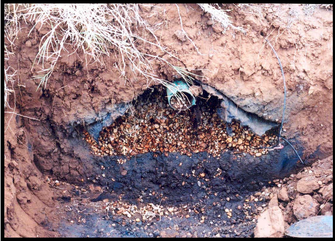
Figure 2.22 View of Biomat at Bottom of Trench 9
