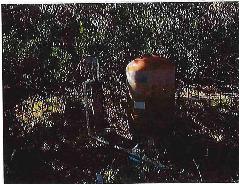
View of well G15 from the east side
