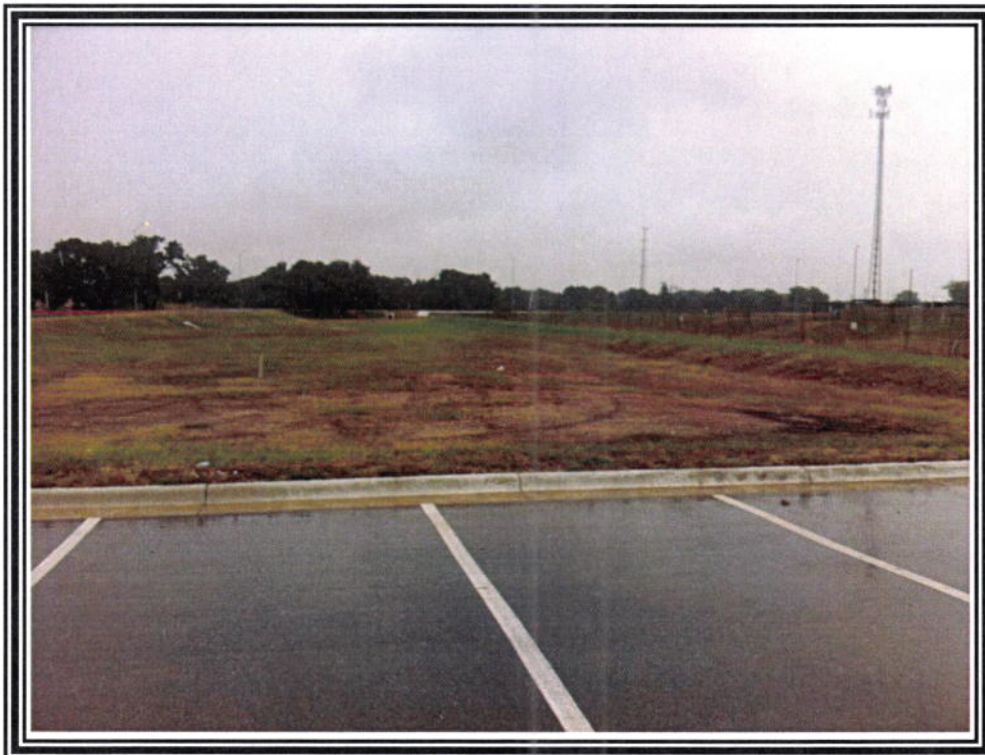
12. View northeast along the north wastewater line from just south of detention pond feature S-1.
