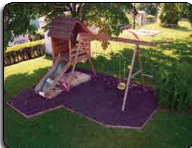
Exhibit 3-3. Loose fill ground rubber installation Photo courtesy of American Rubber Technologies, Jacksonville, FL
